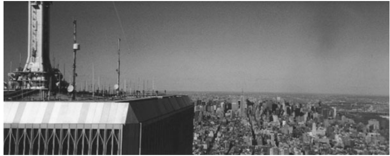
Figure 14.1. Telecommunications infrastructure clustered on the World Trade Center towers.
