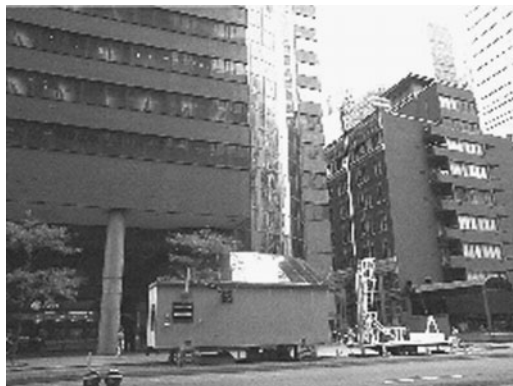
Figure 14.3. A portable cell phone site deployed on Water Street in Lower Manhattan immediately after 9/11.
