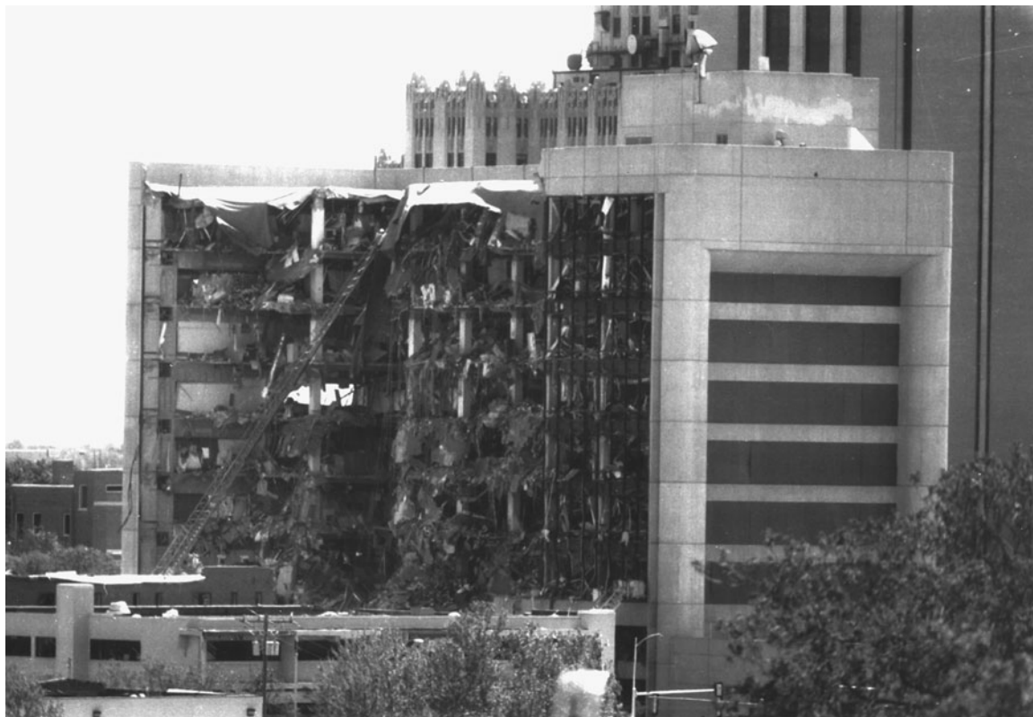
Figure 2.1. The shattered remains of the Alfred P. Murrah Federal Building in Oklahoma City became a grimly familiar image. Courtesy of David Allen, Oklahoma City.
